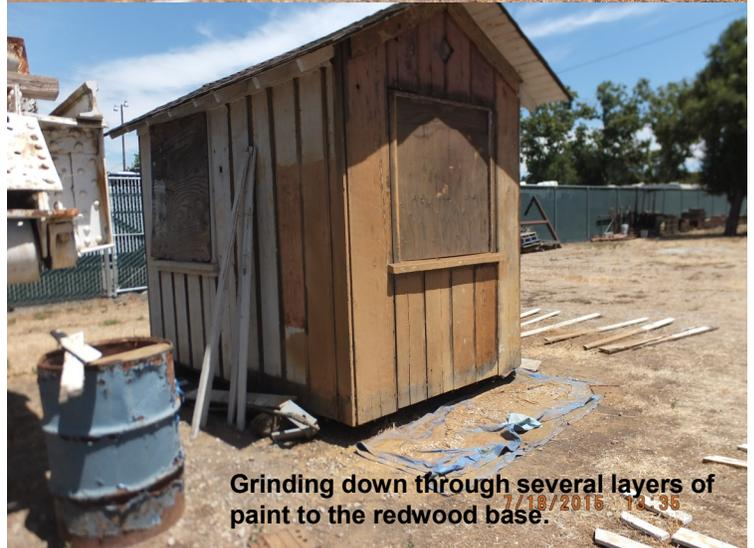
Grinding down through several layers of paint to the redwood base.
