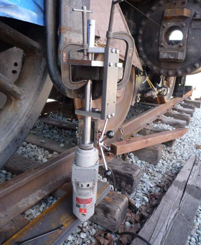
An intricate setup for boring crosshead guide mounting holes.
