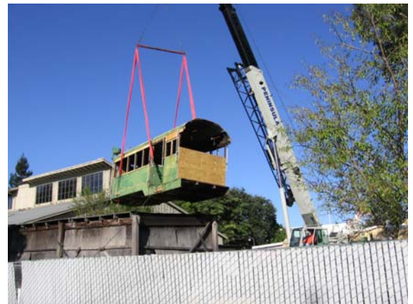
Lifting half body over sheds
