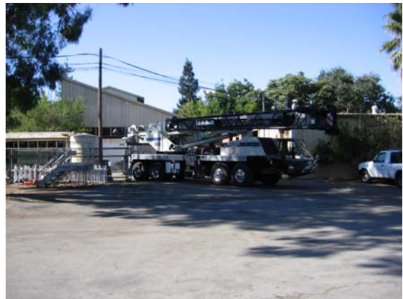
Crane leaving the site
